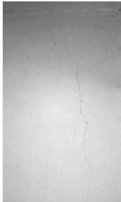
Figure 7: Vertical crack at the centre part of a load bearing wall
