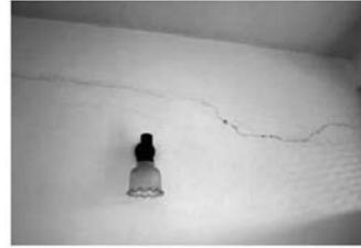
Figure 6: Horizontal cracking under beams
