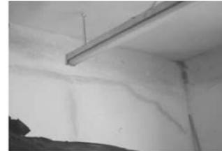
Figure 8: Diagonal crack at the outer edges of concrete framed wall
