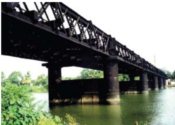
Figure 1: A view of the selected bridge
