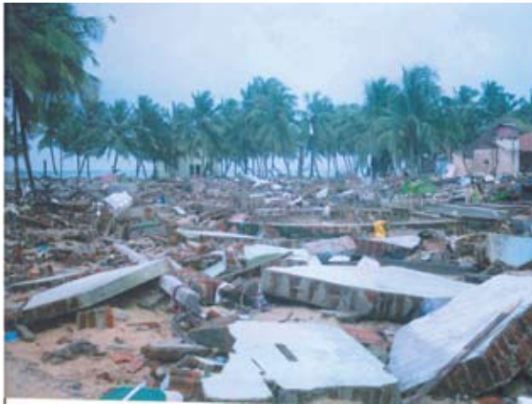
Figure 6: Completely collapsed brickwork structures due to tsunami tidal waves in Kalmunei
