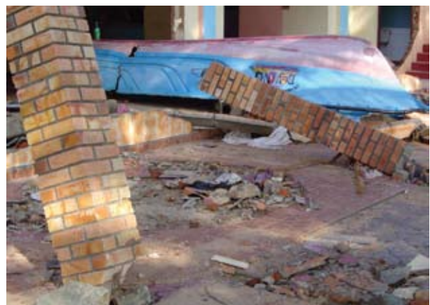
Figure 14: Damage due to a boat taken from tsunami waves
